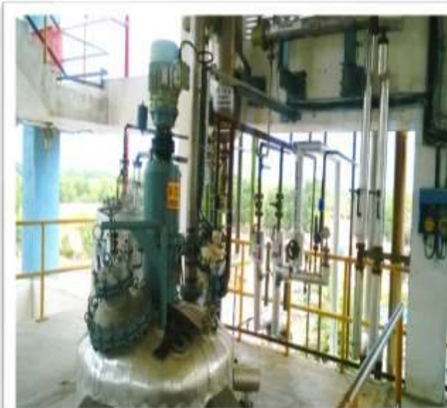
Primary And Secondary Condensers for VOC control
