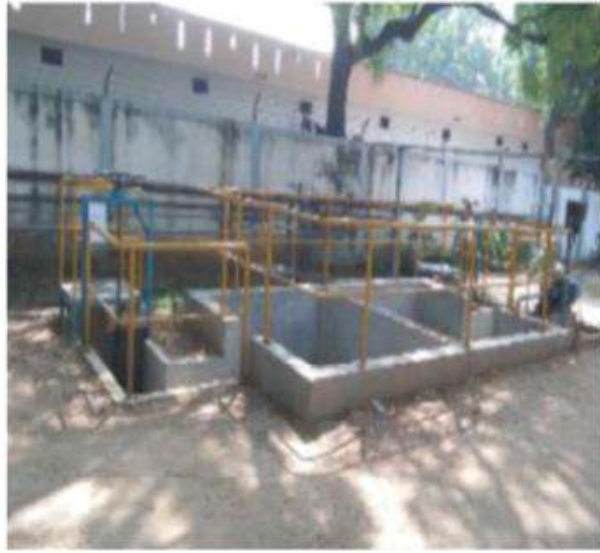
Guard Pond for Storm Drain
