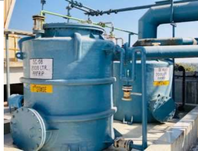
Condenser on Storage tank
