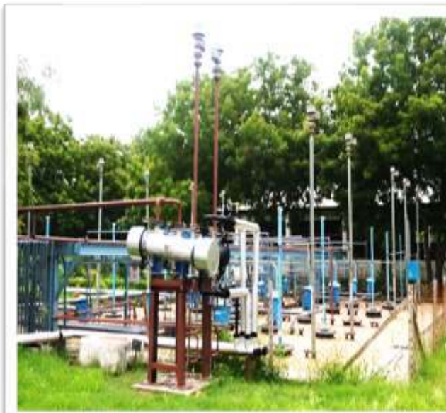
Condenser on Storage tank
