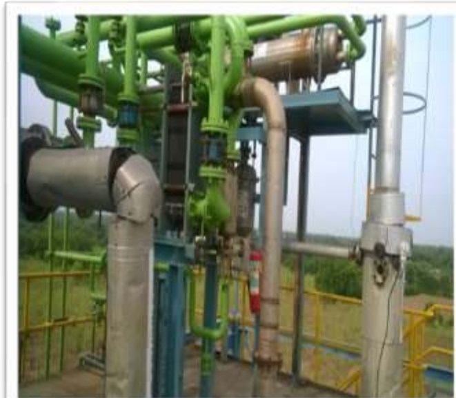
Primary And Secondary Condensers for VOC control
