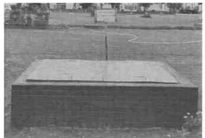
Rain Water Recharge Pit-12
