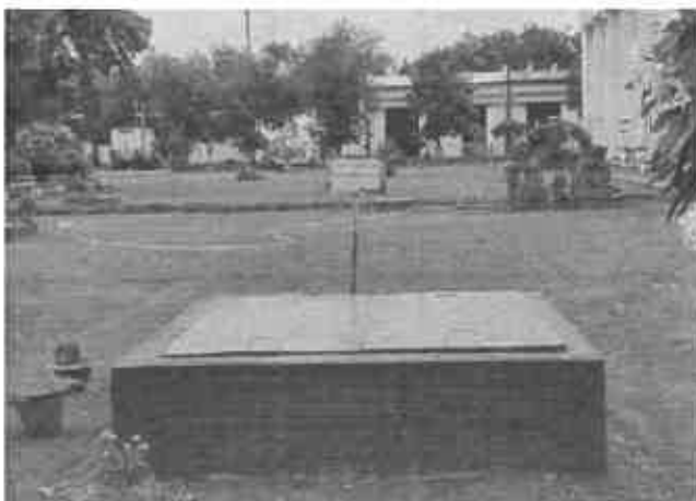
Rain Water Recharge Pit-11
