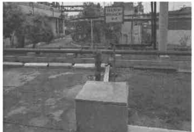
Rain Water Recharge Pit-10
