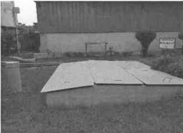
Rain Water Recharge Pit-7
