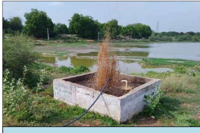
Cleaning & development of recharging borewell
